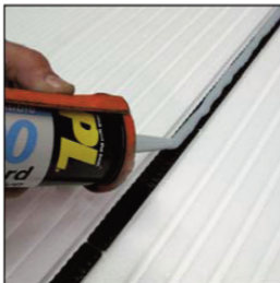
Additional bead of adhesive in corner
