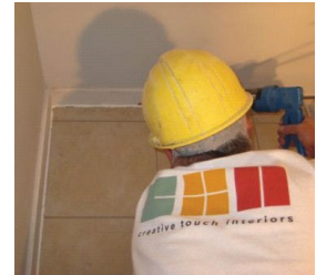
Install perimeter sound isolation strip and fill gap level with a flexible acoustical caulking.
