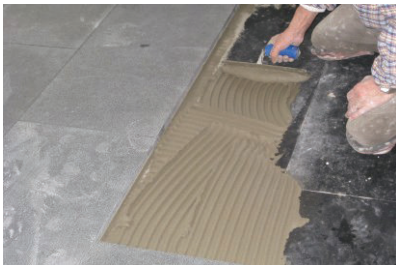
Trowel mortar evenly
