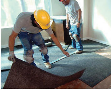
Place one edge of QuietDown HB sheet onto the spread mortar or glue
