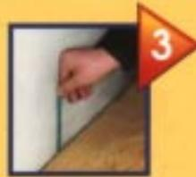
**3** Place the plywood over the entire surface keeping the 3/8" (9 mm) space around the room. Cut where necessary to keep the 3/8" (9 mm) space around any obstacles.
