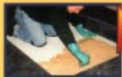
**2** Proceed with the applications of the glue by lifting half of one NeutraPhone™ panel and half of a second panel.
