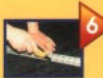
**6** To make the cut, use a knife with a retractable blade or gypsum knife. Do not try to cut the panel in a single stroke. Make two or three passes to get a better result and to avoid injury.
