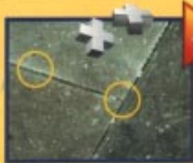
**4** Also leave a 1/8" (3 mm) space between each panel. To be sure that you have correct measurements, use tile spacers.
