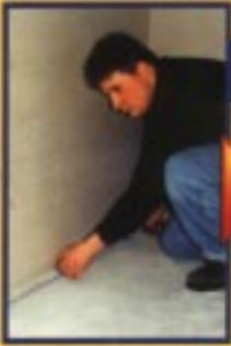
**1** Using a chalk line, trace a line around the room leaving a 3/8" (9 mm) space out from the wall.
