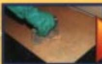
**3** Spread the glue over the whole surface using a 3/16" (5mm) V-trowel. Do not apply too much glue; this will not increase the panel's adherence. any excess glue will cause undulations in the Quiet Floor NP™ and cause problems during the installation of the floor covering. Do the first half of the panel, then the other half. For smaller pieces, take them out completely, apply the glue, and put them back in place. Continue applying the glue under all the Quiet Floor NP™ panels.
