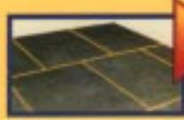
**5** For the second row, cut the first panel in two. Lay it at a distance of 3/8" (9 mm) from the wall and continue the installation to the far end with full-length panels. The end of one panel must always arrive at the center of the panel in the preceding row, as if it were a brick wall. Cut the last panel of the row to the desired length.
